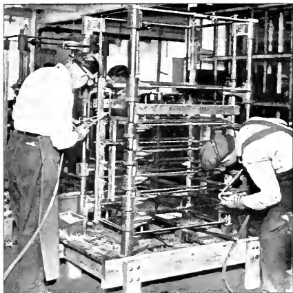
Welding the frames of Simmons steel furniture. All welding is done in special jigs so that parts are interchangeable.
